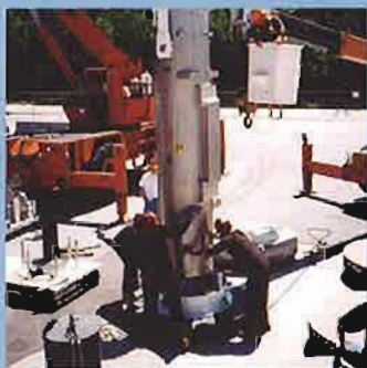
Intermediate level waste inserted into in-ground storage containers at the WWMF
