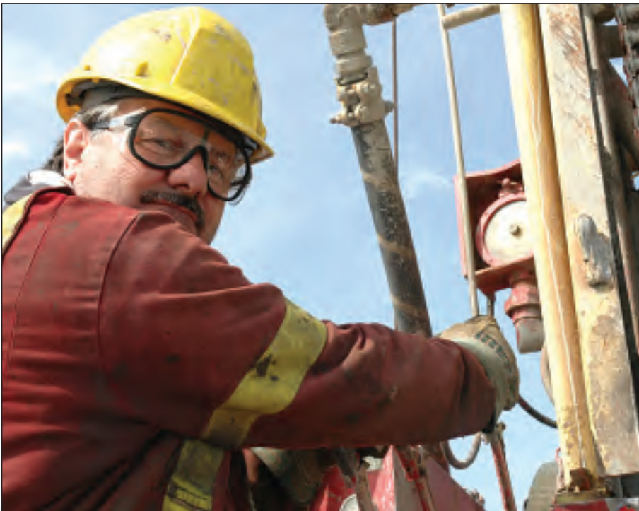
Driller Paul Marier is hard at work at the Bruce site where Phase Two of the geoscientific site characterization plan for OPG's proposed DGR, which includes the drilling of two vertical boreholes at two separate drill sites, began at the end of March.
