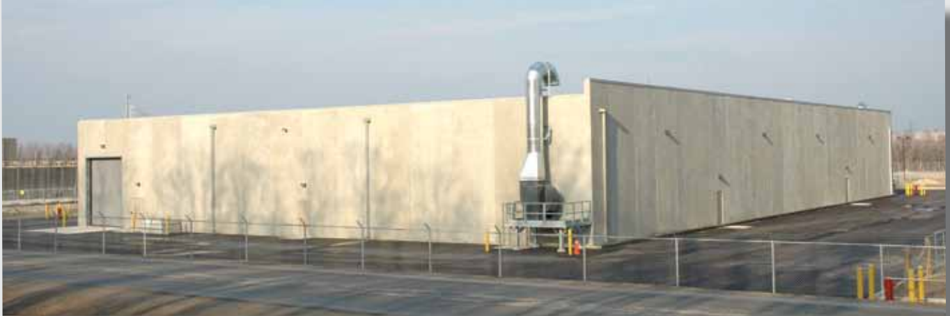
The WWMF is ready to receive Bruce Power refurbishment waste from Bruce A units 1 & 2 with the construction of two new storage buildings.
