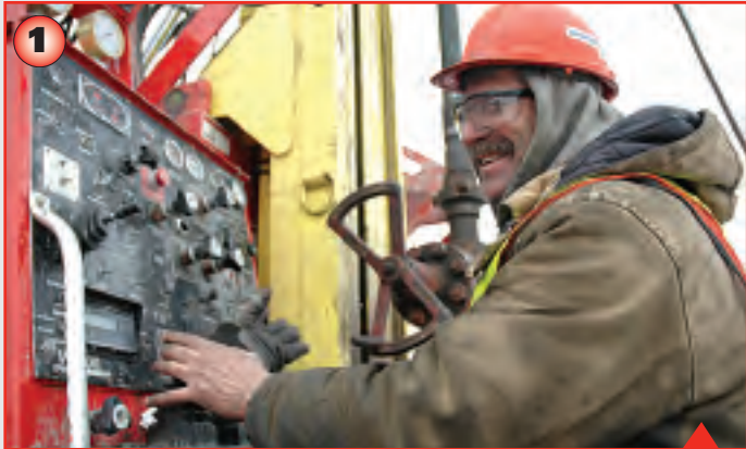
1. Doug Fenton of Davidson Drilling Limited of Wingham operates the controls of the Drill Rig, currently coring on site at the WWMF, on a 24/7 basis. Drilling and coring of the two boreholes DGR 1 and DGR 2 will be completed in the summer months. At that time, a number of geophysical and hydraulic tests will take place within the boreholes to gather more information about the properties of the formations. When this testing is complete, multi-level groundwater monitoring equipment will be installed in both boreholes to provide a baseline of information on the different groundwater systems located in shallow, intermediate and deep regions.
