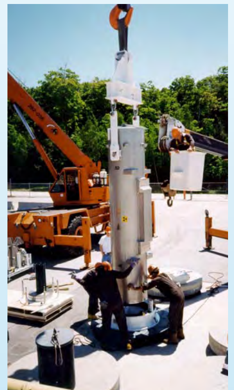
Ontario Power Generation staff carefully lower intermediate level waste into an in-ground storage container
