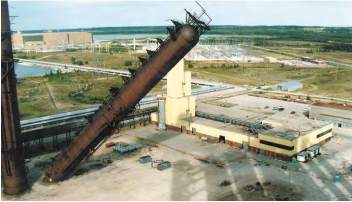
These two photographs provide an excellent visual of a "tower drop". They show a heavy water tower from enriching unit 8 being dropped in 1995. The last two sets of Heavy Water Plant towers are scheduled to come down in 2005.
