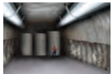
Intermediate level waste emplacement room.
