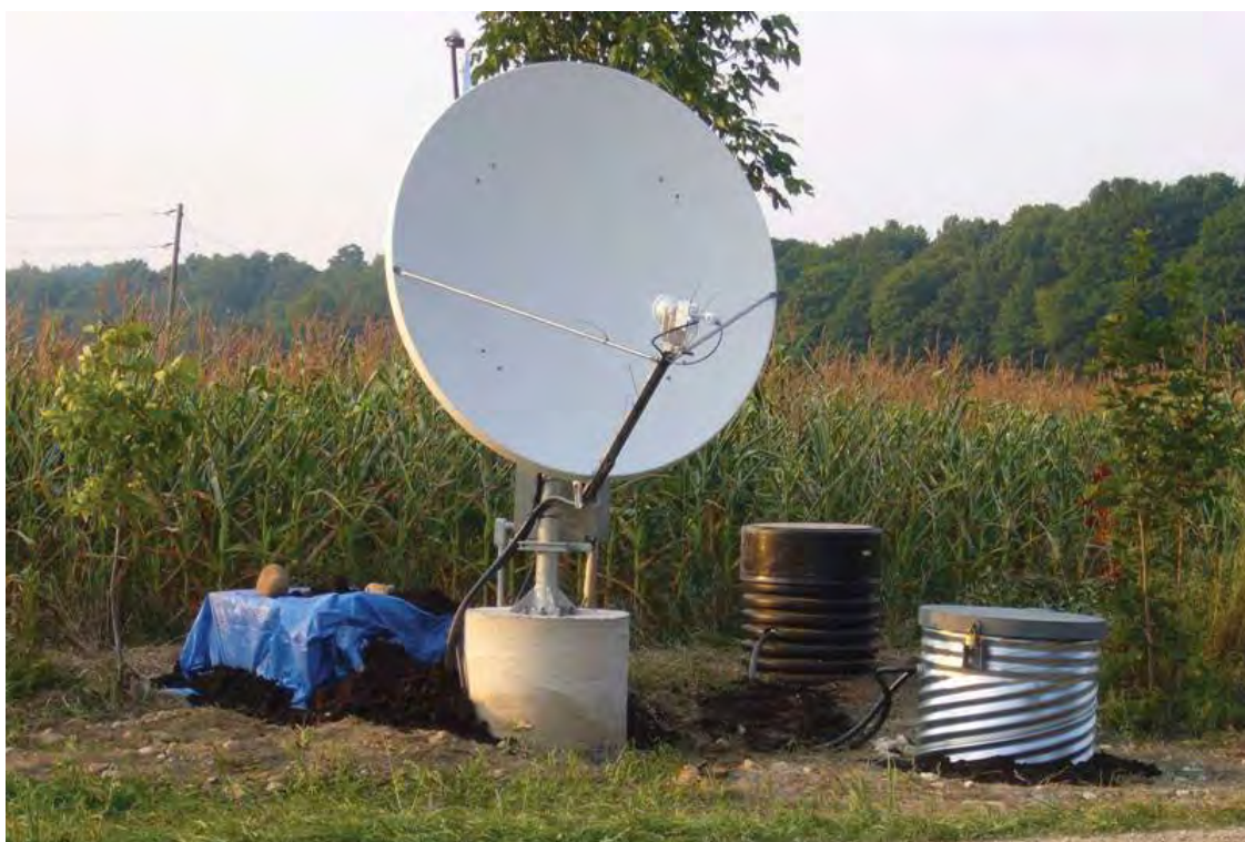
Low level seismic monitor
