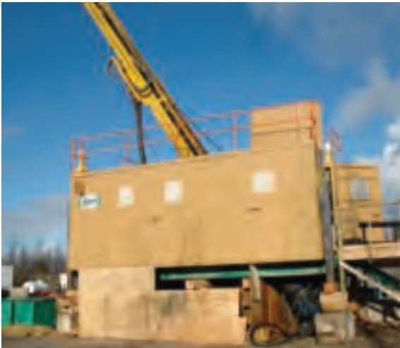
Above: Inclined drilling verifies the nature of vertical bedrock structure and its effect on L&ILW DGR implementation.
