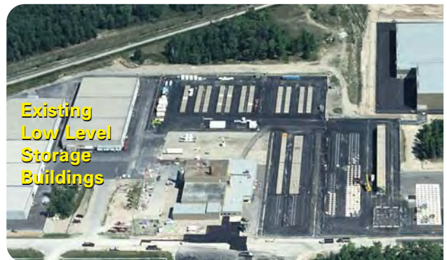
The proposed new LLSBs are to be constructed adjacent to the existing LLSBs at the WWMF
