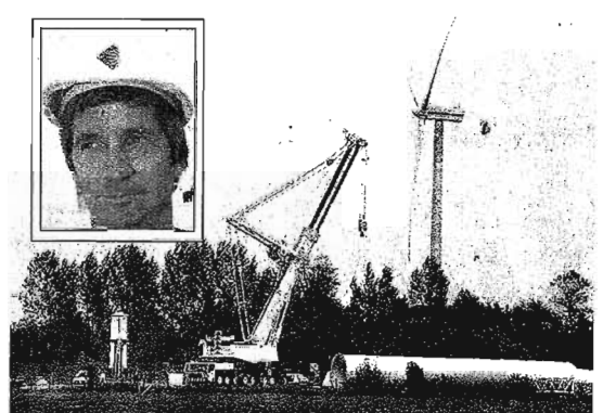
Glen Estill, inset at the site of Skygeneration's new turbines during construction last fall.
