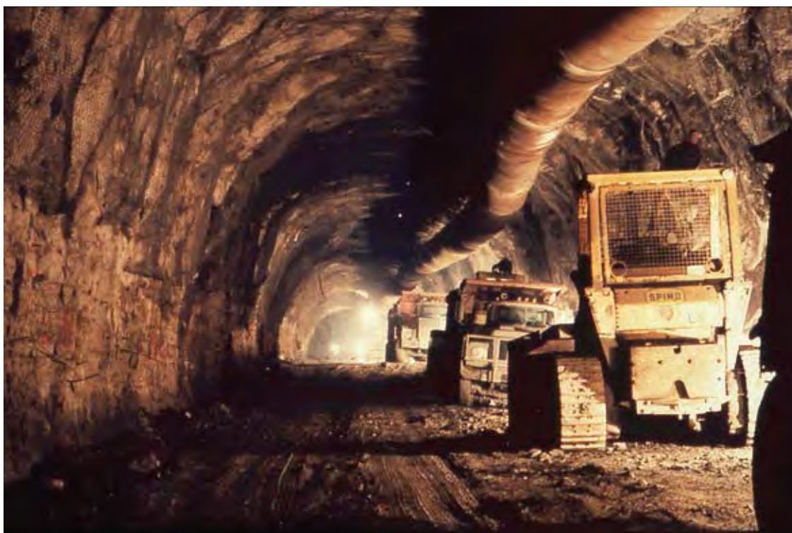
Construction during Darlington cooling water intake tunnel
