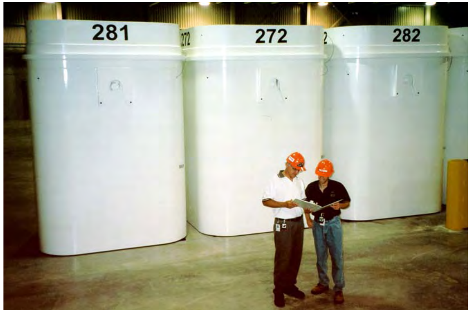
Gary Varsava (left) Responsible System Engineer, and Mark Billington Section Manager Western Used Fuel Dry Storage, perform a check in the Storage Building.
