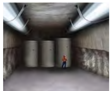
3: Resin Liner Shields within ILW emplacement room
