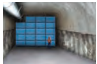
Low level waste emplacement room.
