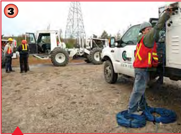
3. A seismic cable is plugged into the recorder truck (doghouse) so data can be transmitted to seismograph.
