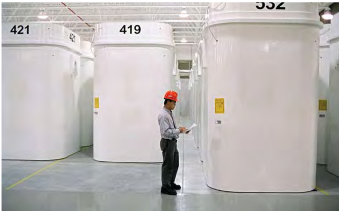
Used fuel dry storage containers
