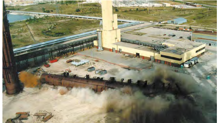
These two photographs provide an excellent visual of a "tower drop". They show a heavy water tower from enriching unit 8 being dropped in 1995. The last two sets of Heavy Water Plant towers are scheduled to come down in 2005.
