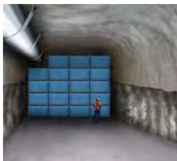
2: LLW emplacement room
